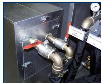
Option: ips-PWS 100 Hot water design up to 95°C
